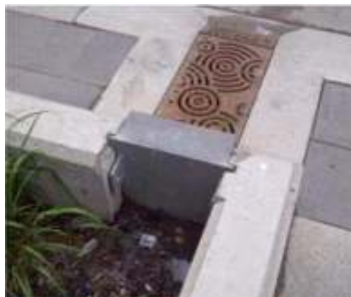
Figure 4.2.7.1: Inlet gate to prevent chloride loading during winter months
