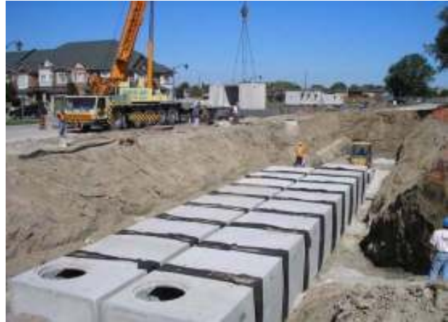
Rainwater harvesting systems can range from widely distributed small scale practices such as residential rain barrels to large subsurface units as shown above.
