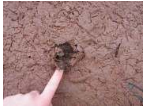
Figure 8.1 – Clay sediment accumulated on top of the mulch layer of a bioretention facility resulting from improper erosion and sediment controls.
