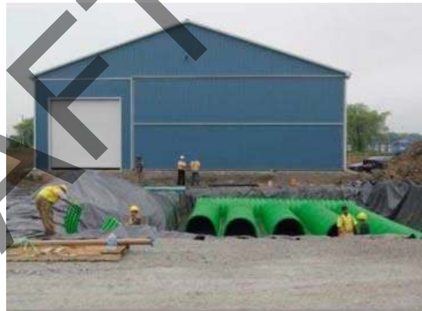
Infiltration chambers can be installed below conventional parking surface without compromising
