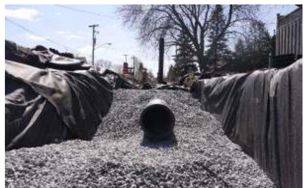
Perforated pipe systems employ many of the same materials and construction practices as conventional storm sewer pipes.
